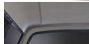
Fiberglass Finish Interior
